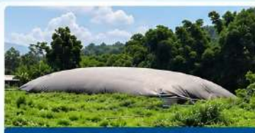
Large Farm Biogas Digester
